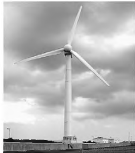
Fig. 11 Japan's first 2 000 kW wind turbine (MWT-S2000 at Gushikawa Power Station, Okinawa New Energy Development Co.)
